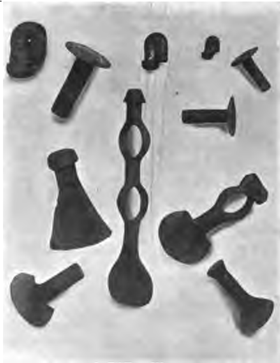
FIG. 28.— Forge Tests for Rivets.
